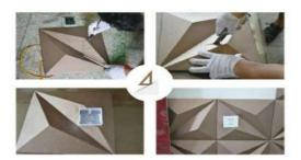
When there is outlet, measure the position on the panel and Cut. Then put the inner box in the hole, cover the outlet.
