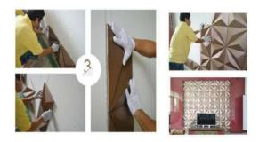
Apply the first panel on the lined bottom middle position, Then go ahead with the Neighbour panels by the same way. When applying on the Wall, press a little bit for around 15 seconds to make sure of no gap between. When the size of the wall won't match The panels, cut the panels by utility knife as need.
