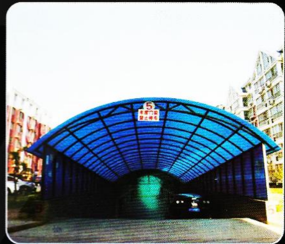
Garage Entrance Roof
