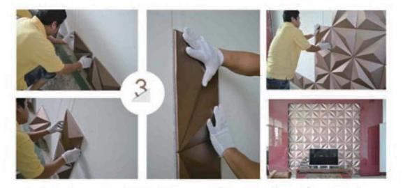
Apply the first panel on the lined bottom middle position, then, go ahead with the neighbour panels by the same way. When applying on the wall, press a little bit for around 15 seconds to make sure of no gap between. When the size of the wall won't match the panels, cut the panels by utility knife as need.
