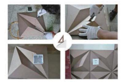
When there is outlet, measure the position on the panel and cut. Then put the inner box in the hole, cover the outlet.
