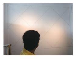
STEP 2: Refer to the panel size, measure and mark each unit on the wall
