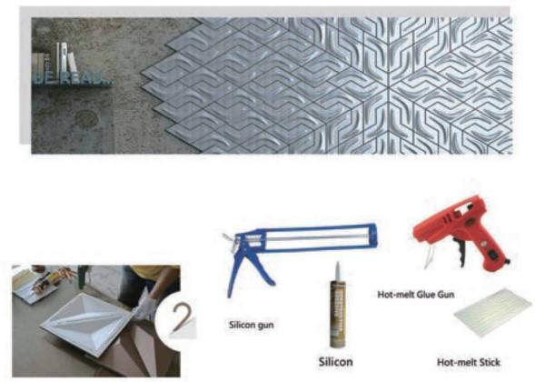
Prepare the tools and materials as pictures. Apply the silicon on 4 corners and middle on the back of panel. Then, apply the Hot-melt glue on 4 corners.
