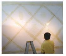
STEP 3: Brush the contact glue on the marked lines and in the middle of each cell
