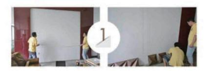
Make sure the surface of the wall is clean. For lime wall, please paint with a coat of latex. Square off the wall according to the size of panels.
