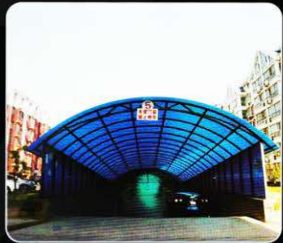
Garage Entrance Roof
