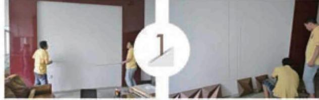
Make sure the surface of the wall is clean. For lime wall, please paint with a coat of latex. Square off the wall according to the size of panels.
