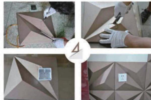
When there is outlet, measure the position on the panel and cut. Then put the inner box in the hole, cover the outlet.
