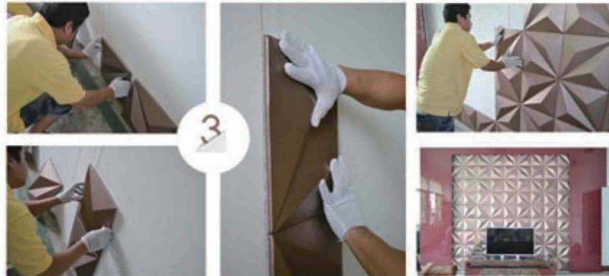
Apply the first panel on the lined bottom middle position, then, go ahead with the neighbour panels by the same way. When applying on the wall, press a little bit for around 15 seconds to make sure of no gap between. When the size of the wall won't match the panels, cut the panels by utility knife as need.
